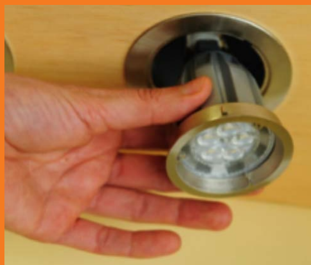
Halogen replacement with LED
